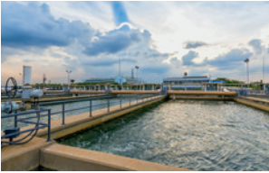
Collecting and retaining basins
