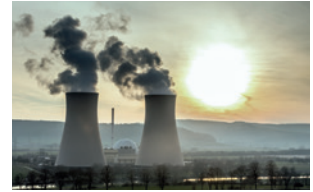
Power station cooling towers
