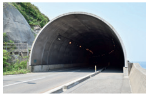
Tunnels and concrete pipes
